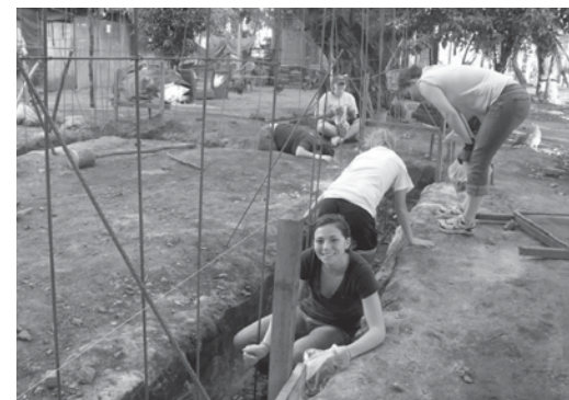
Emily Busby joins others working in the trenches.
